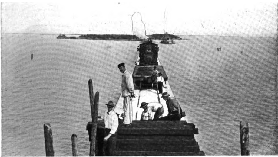
Work train on Long Key Viaduct, Long Key in the distance.
